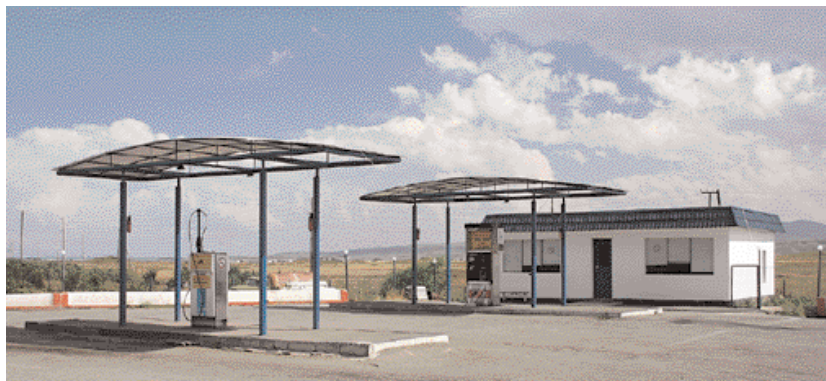
Refuelling station in Sevan city
